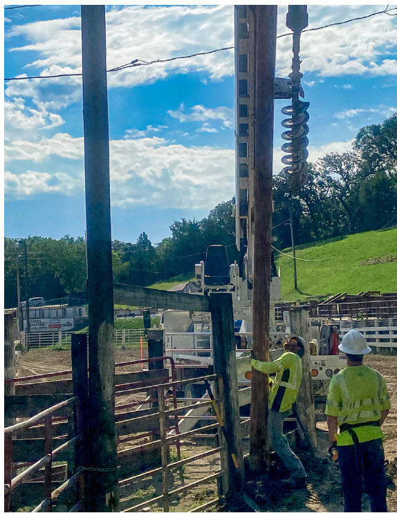
Jefferson linemen setting a pole at the Dayton Rodeo Arena
